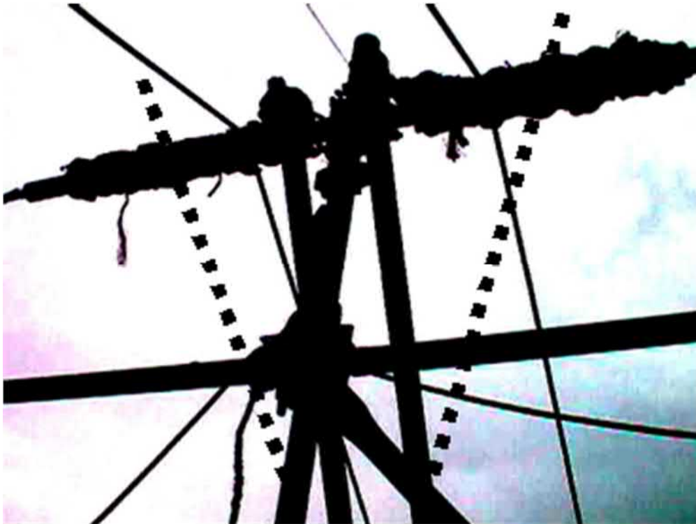
Figure 24 Cantilevered Hawser Structure (Non-compliant)
