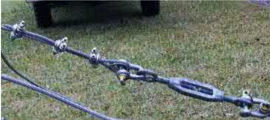
Figure 37 Turnbuckle Hawser Base Clamp Tensioning
