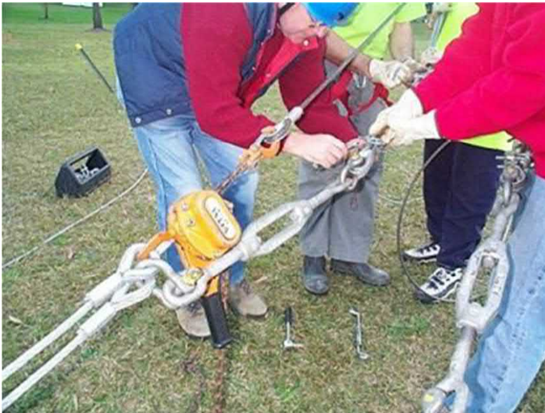
Figure 39 Cum-along Tensioning System
