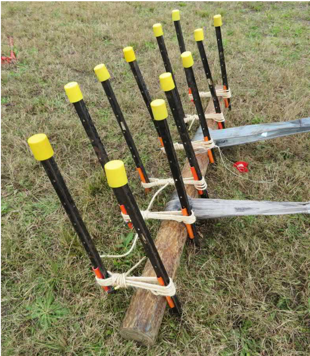
Figure 15 Log and Picket Anchor
