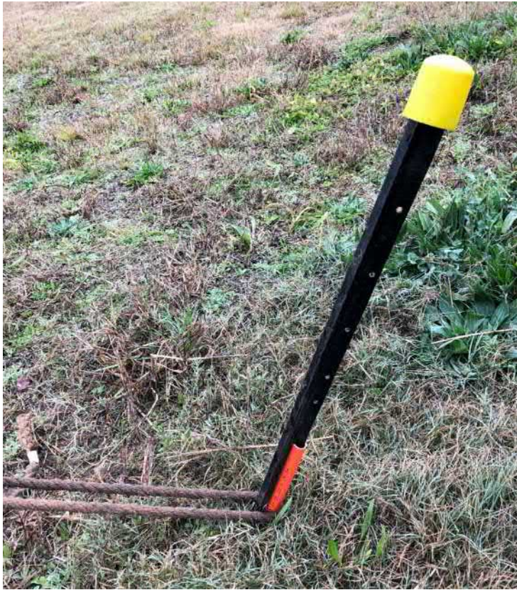
Figure 22 Picket Fibre Rope Protection
