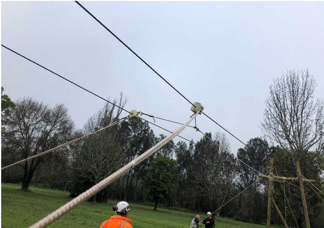
Figure 32 Double Hawser Dynamic Brake
